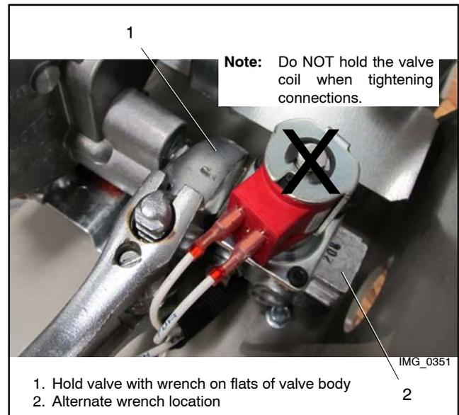
Figure 1-8 Holding Fuel Valve to Tighten Fuel Connections
